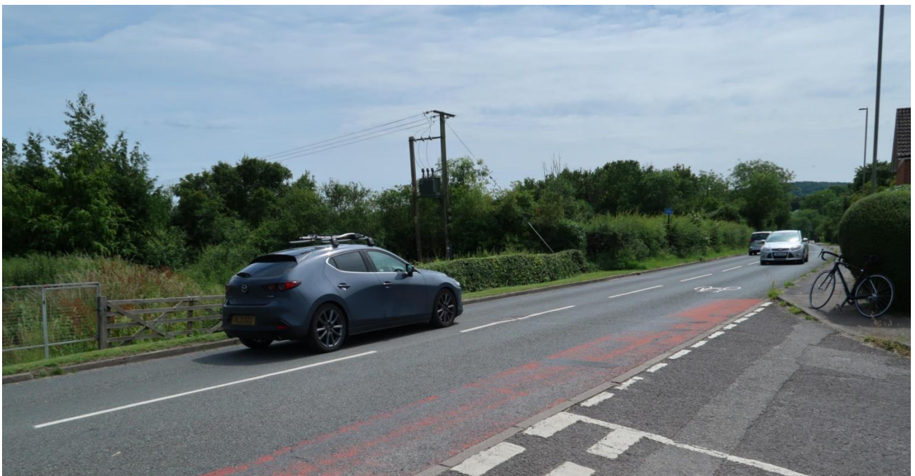
Figure 2: view of the Causeway near SDA8 looking south. Both photographs were taken on 14 June 2026.
