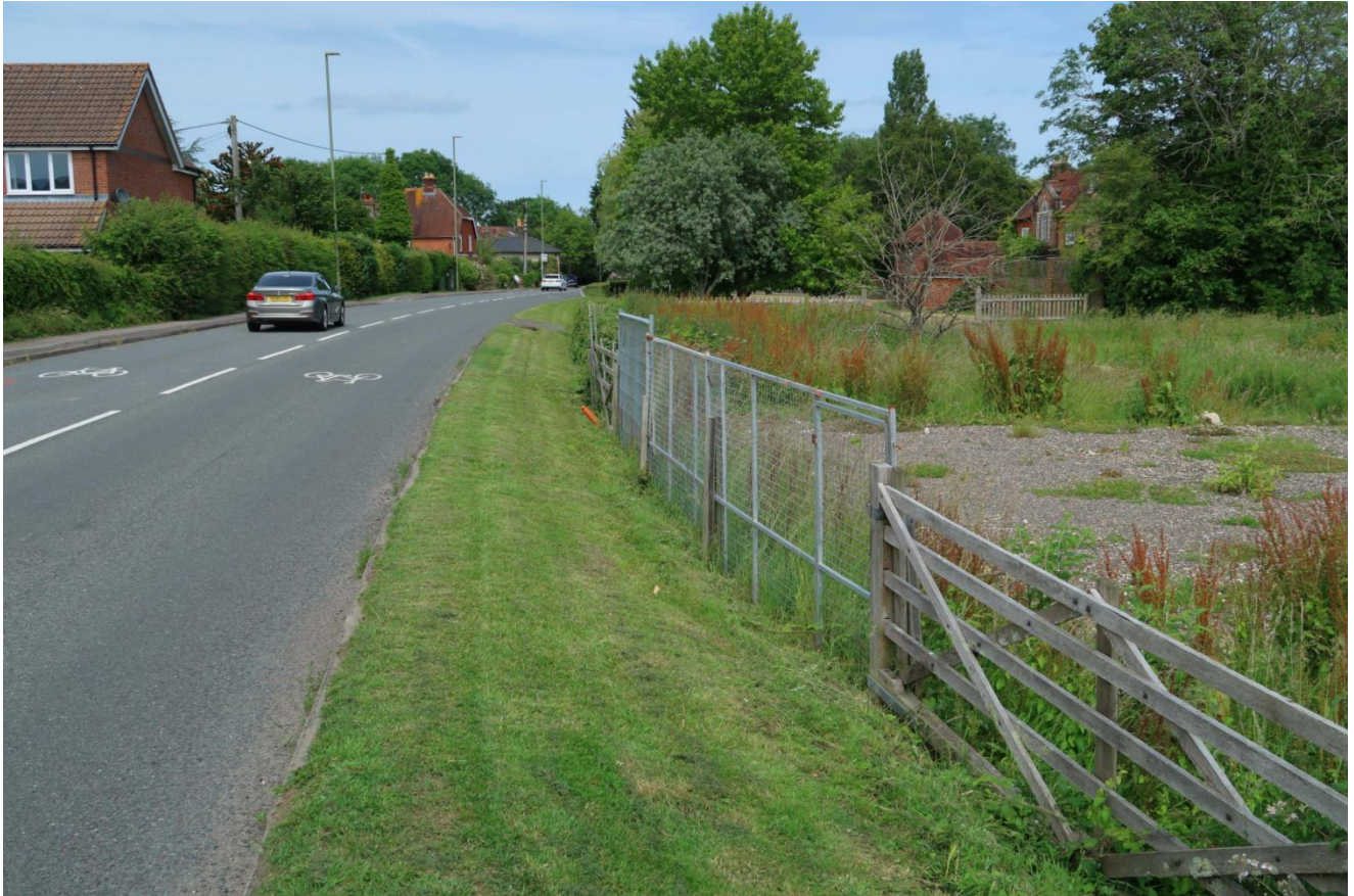
Figure 1: view of the Causeway near SDA8 looking north. The surface makings on the carriageway indicate that pedal cycles should use the carriageway.
