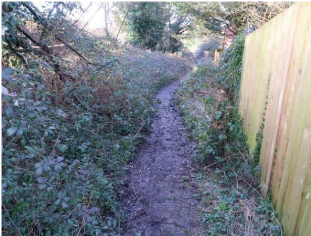
Figure 6: PROW 189/44a/2 where it runs parallel with Nos 120-124 Borough Road. Brambles and mud render this route impassable for most journeys.
