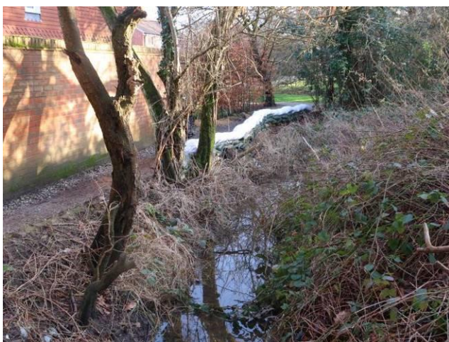
Figure 8: PROW 189/42/1 behind near No 6 Reed Way. Note the sandbags used to mitigate a flooding issue.
